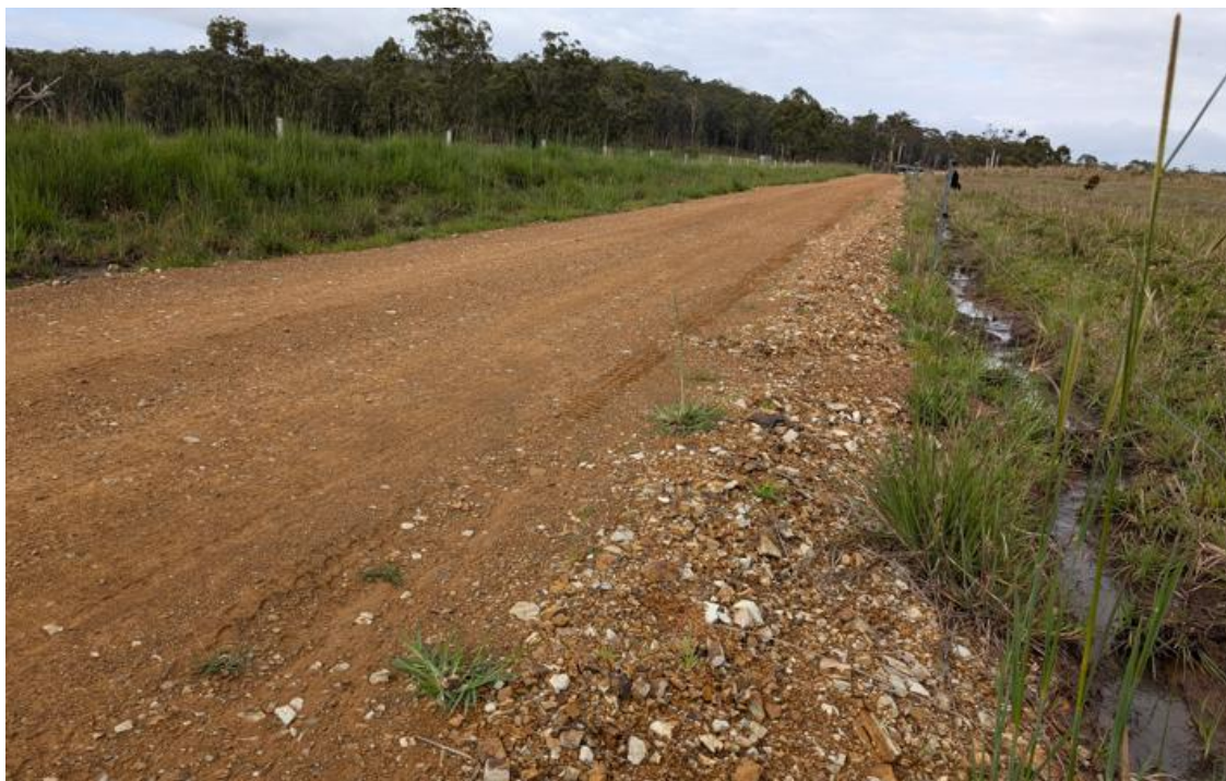
Plate 3.3 – Existing gravel access track, near property entrance.
