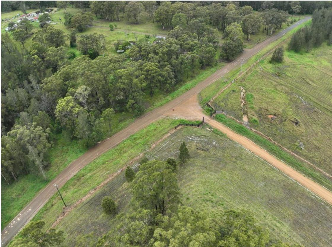
Plate 3.2 – Oblique aerial drone image of driveway off Shallow Bay Road (view in easterly direction).
